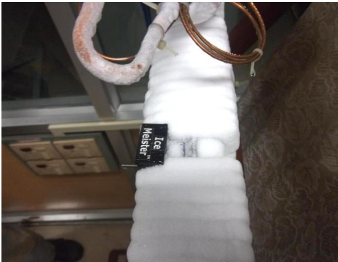
Figure 2 -- 9734 installs directly on evaporator coil assemblies
